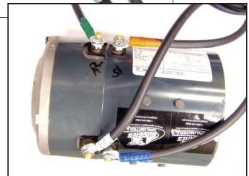
15. Orange Cable Installation
